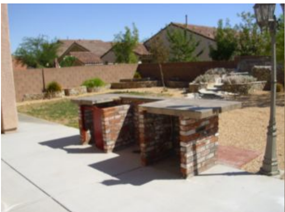
Grilling area with no equipment installed
