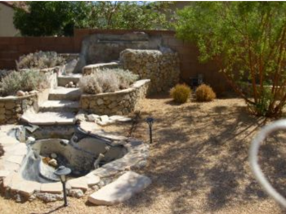
Inoperable water feature
