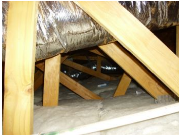
Typical attic insulation
